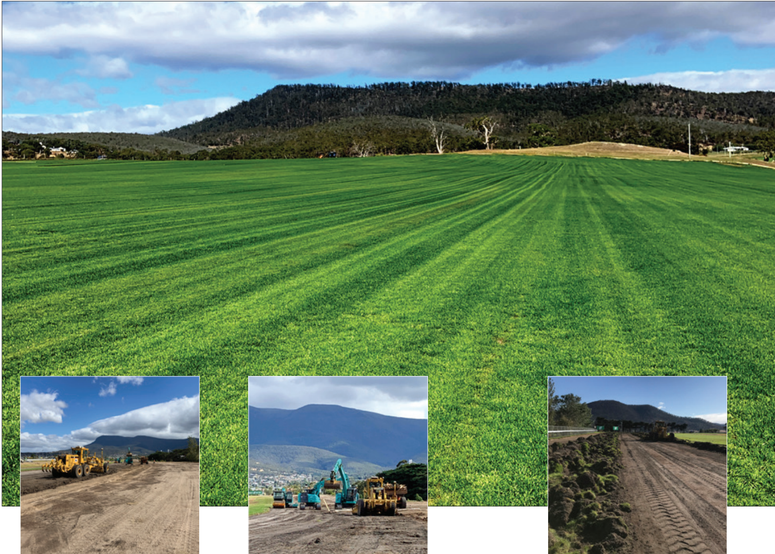
Images: (Main) New turf being grown at StrathAyr Turf Farm at Richmond in readiness for laying of the Elwick track. (Inset) Stage 1 work in progress at Elwick.
