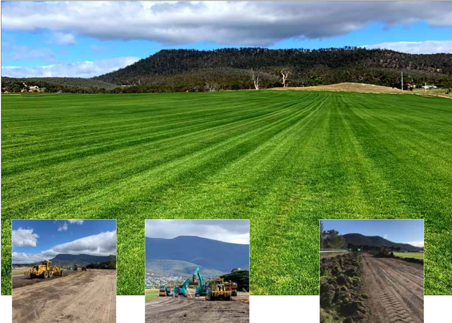
Images: (Main) New turf being grown at StrathAyr Turf Farm at Richmond in readiness for laying of the Elwick track. (Inset) Stage 1 work in progress at Elwick.
